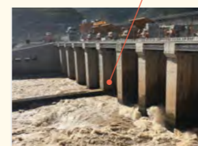
Xayaburi dam (1,285 MW)
