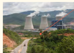
Hongsa lignite power plant (1,878 MW)
